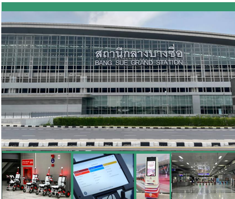
Exhibit 22: Bang Sue Grand Station. © Office of Transport and Traffic Policy and Planning
